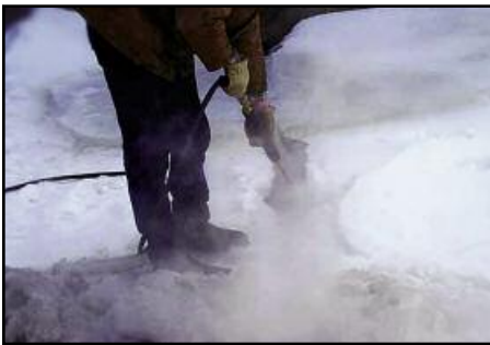
(Breaking Ice Dam)
